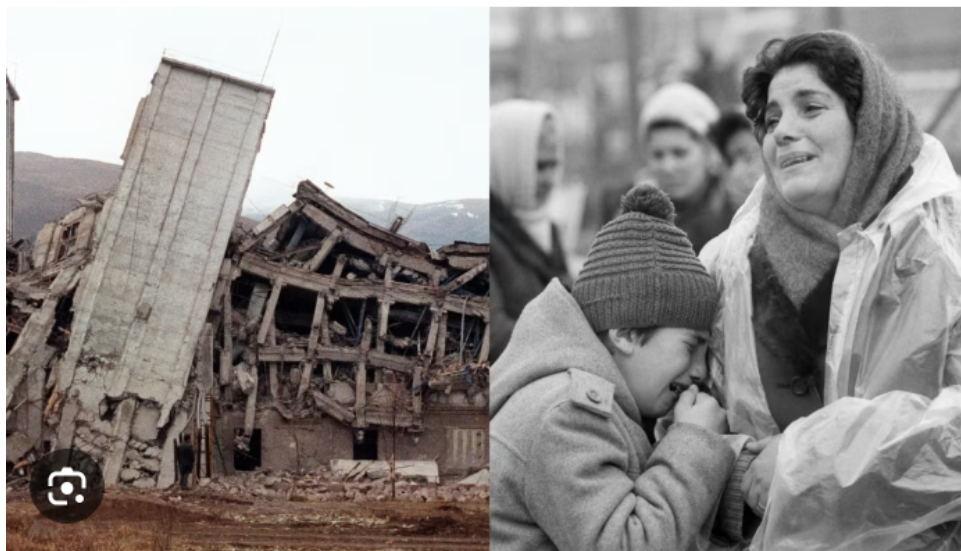
Figure 3.B2: Note: This picture illustrates episodes from the 1988 Armenian Earthquake.
